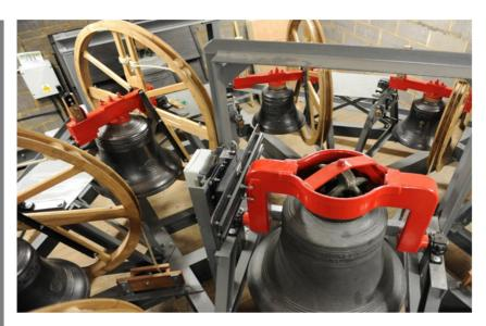
NEW PEAL OF EIGHT IN RADIAL FRAME TOGETHER WITH ELECTRICALLY SWUNG BOURDON AND STATIONARY SERVICE BELL, SOUTH OCKENDON.
