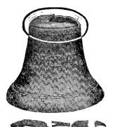
A large Bell fractured at dome and parts completely broken out.
