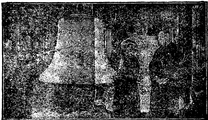
YORK MINSTER : Hoisting one of the Bells into the SW Tower
